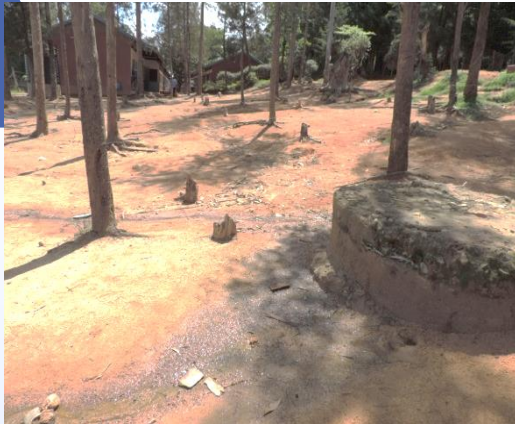
Spillage from the septic tank – both the septic tank and the pit latrines are full
